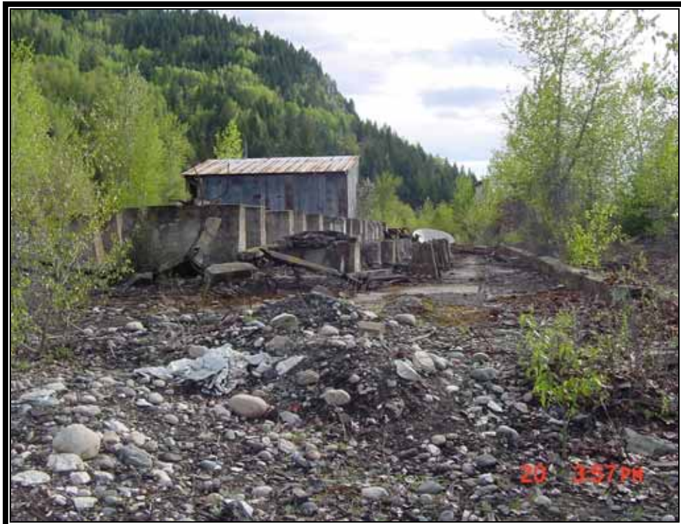
Photo 4. Remaining foundation on-site
