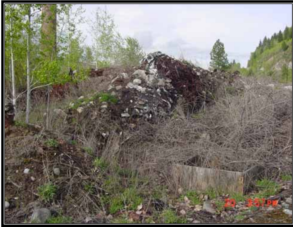
Photo 3. Remaining foundation on-site
