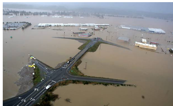
A 2007 flood completely submerged I-5 in Lewis County and damaged several area water systems. (Photo courtesy of Washington Department of Transportation.)
