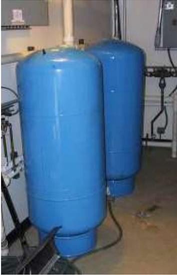
Chapter 5 explains how to make well pumps and pressure tanks work together as a single system capable of reliably providing safe drinking water to customers of new Group A-TNC water systems.
