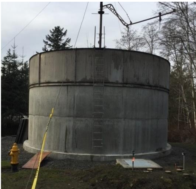
Construction of a new tank.
