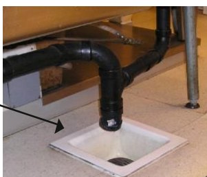
Indirect Drain at a food preparation Sink
