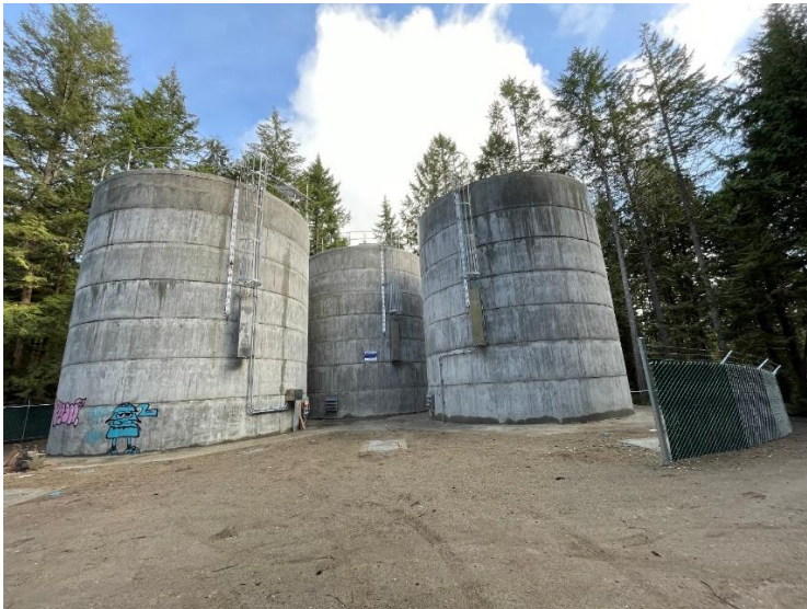
Concrete storage tanks to provide additional capacity for the customers.
