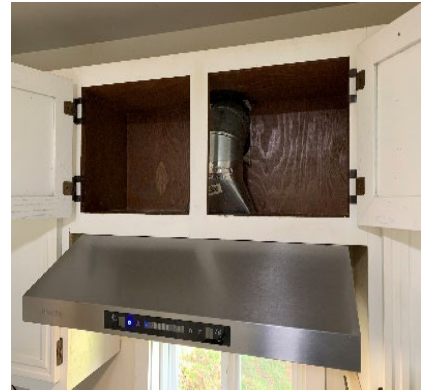
A ducted range hood (above) ideally sends air outside. A recirculating range hood (below) does not send air outside.
