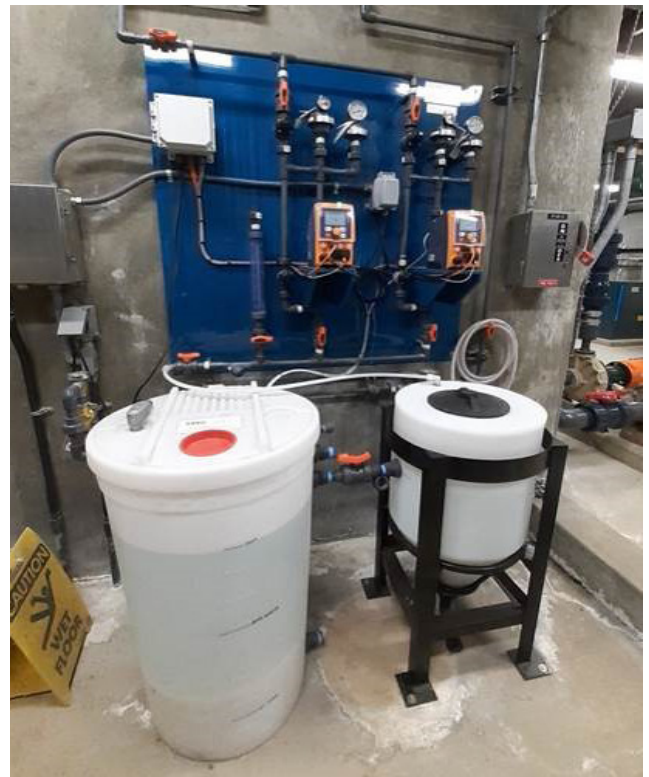
Example of a secondary day-tank in use.
