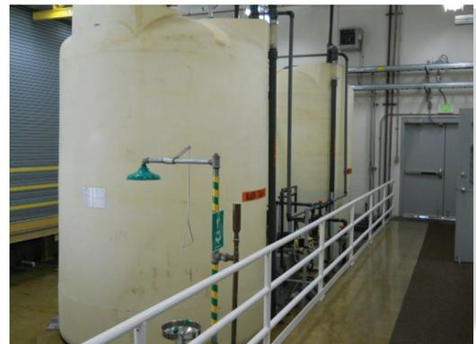
*Bulk sodium hydroxide storage tank with containment and eyewash station.*
