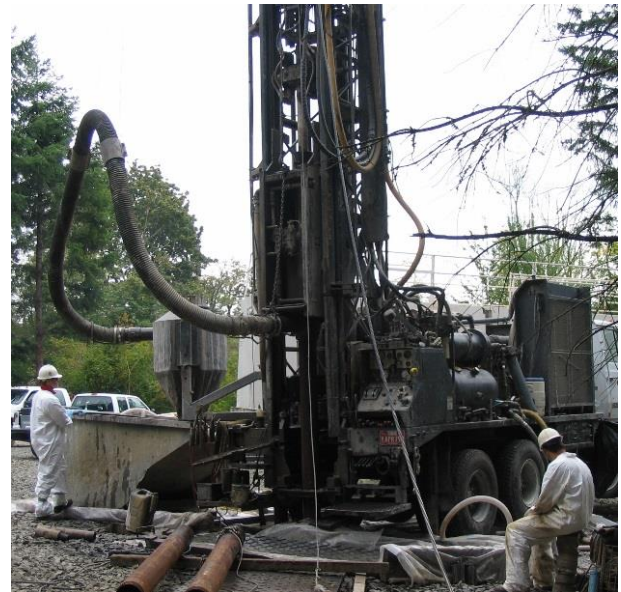
Wells drilled near Landsburg Mine help us understand how waste inside the mine impacts groundwater.
