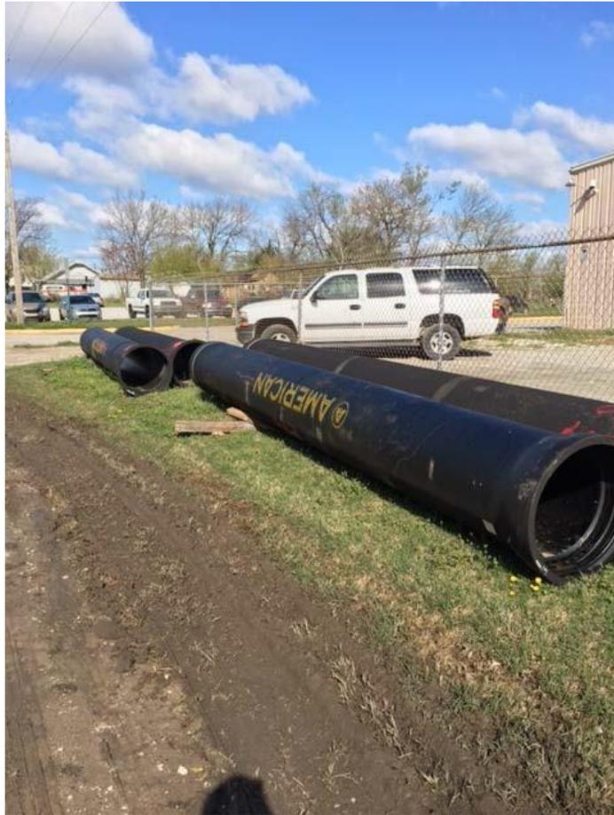
Ductile iron pipe for a raw water line to a new water treatment plant in Arkansas City, KS.
