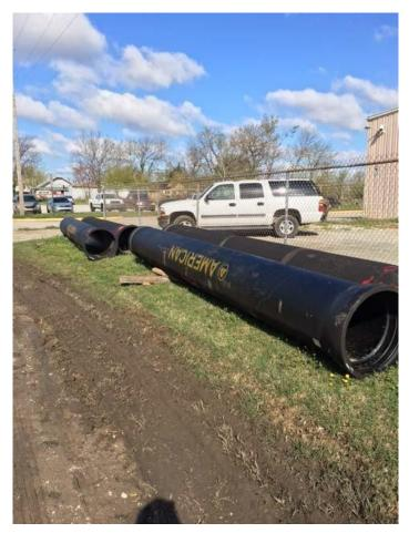
Ductile iron pipe for a raw water line to a new water treatment plant in Arkansas City, KS.
