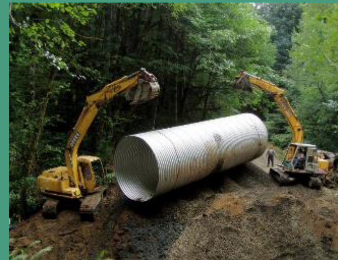
Culvert installation
