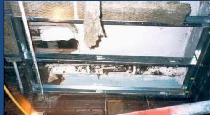
Damaged asbestos pipe insulation
