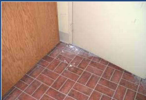
Asbestos debris on floor
