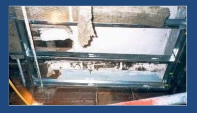
**Damaged asbestos pipe insulation**
