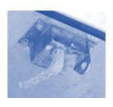
Operators are experiencing problems with some commercially available hatches that are generally very well constructed. Most are made of stainless steel. However, the internal rods, locks, screws, and connectors are not. These eventually rust and break under the constant corrosive conditions. Broken latches must be replaced or removed. Replacement parts may not be available. Cement blocks may be needed to hold down the lid. Locks need to be reinstalled.
