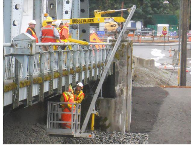
*Installing 320 feet of pipe under the Snohomish County Bridge #15 on Dubuque Road was a challenging part of the project. Workers had to drill through the concrete to install a 12-inch iron pipe, and then hang a 16-inch steel wrapped polyethylene pipe on supports. After installing the pipes, the roadway was restored to its original condition.*
