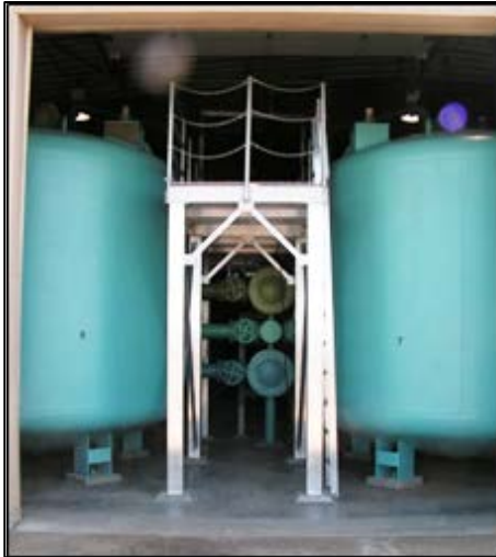
Prosser added green sand pressure filters to increase its capacity.
