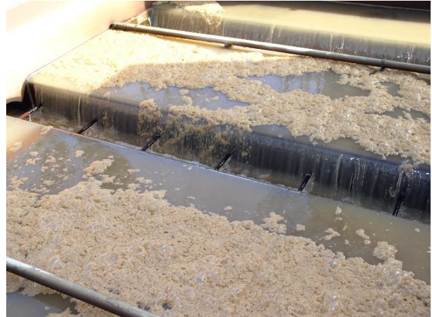
Backwashing a rapid-rate filter.
